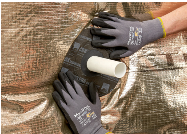
Fix grommet around pipes and ducting
