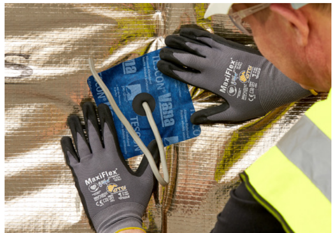
Fix grommet around electric wiring
